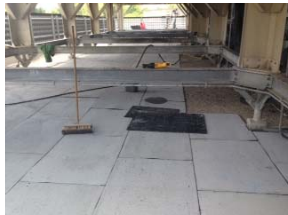
Finished Roof with Walk Mats in Place
