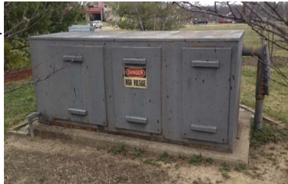
Current ‘Pad Mount’ Loop Switch
