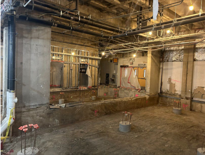
Left: Nunn Hall first floor – new structural piers, looking toward elevators. Right: new 5 th floor restroom. Early October 2024
