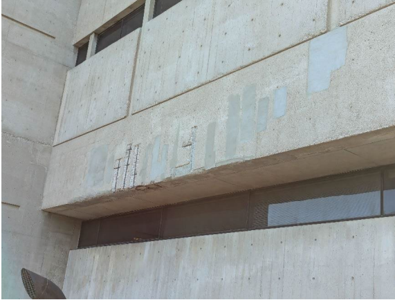
Repairs, patching and cleaning underway on Nunn Hall
