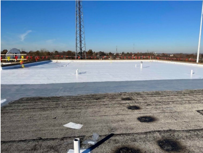
Campbell Hall Roof Restoration Underway
