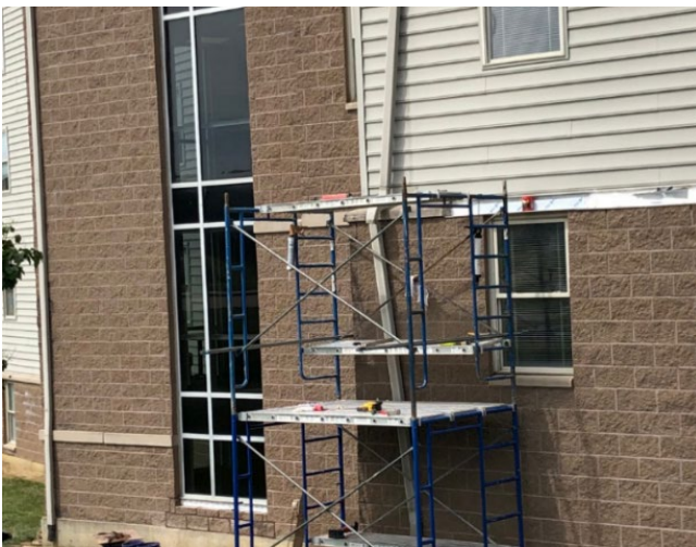
Façade Repairs Underway at University Suites
