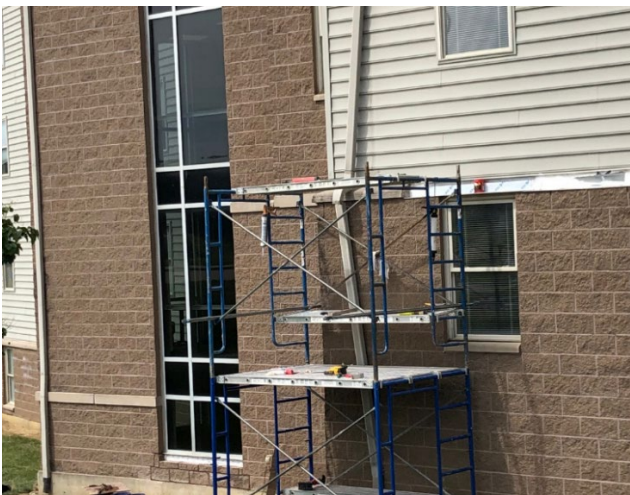
Façade Repairs Underway at University Suites
