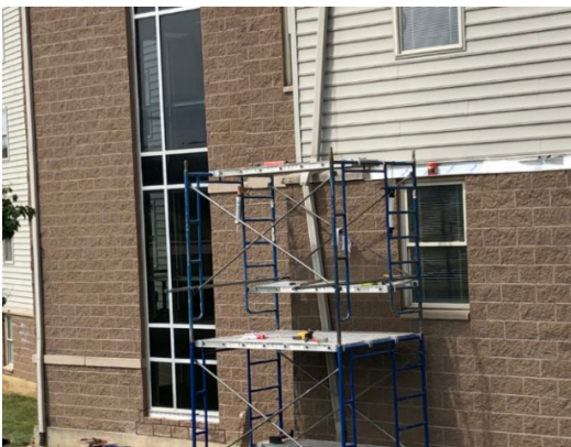
Façade Repairs Underway at University Suites
