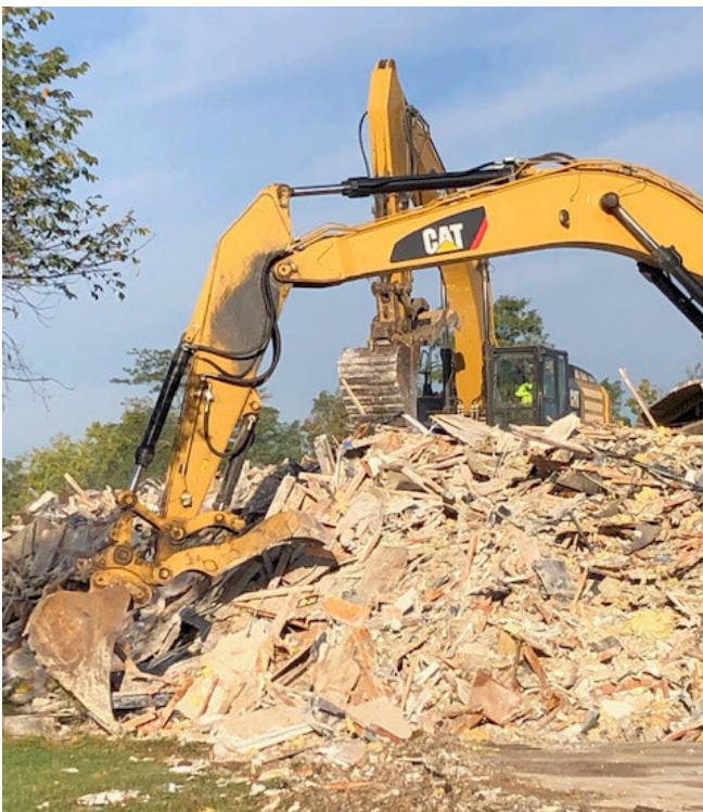
Demolition of Oak Hall, October 1, 2021
