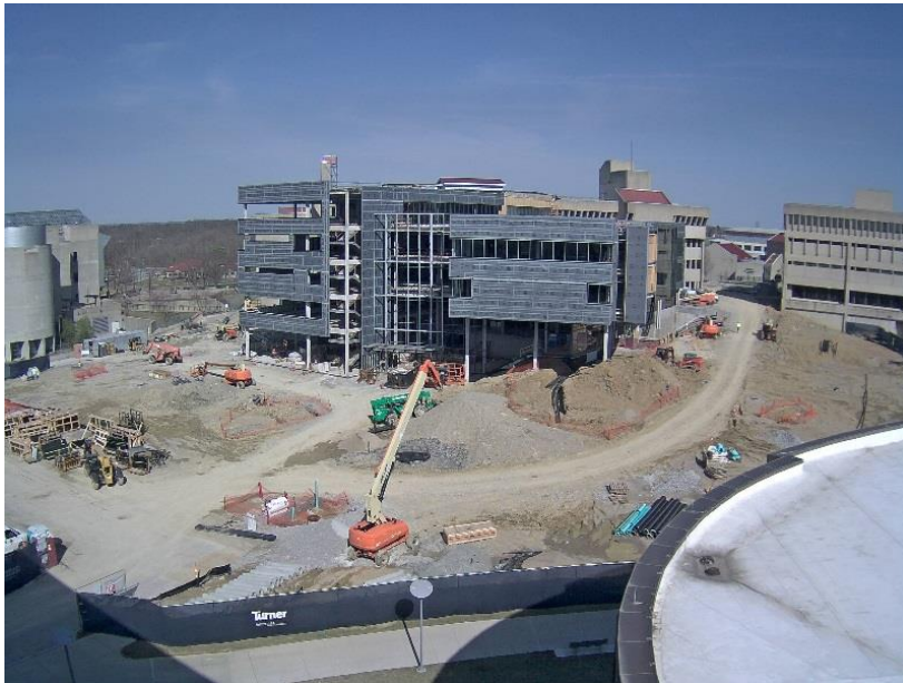
Webcam Photo of Construction Site
