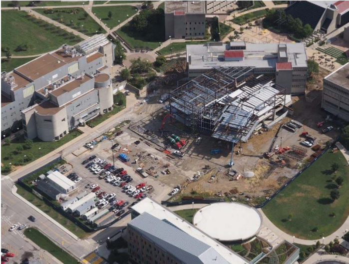
Aerial Photo of Construction Site - 1
