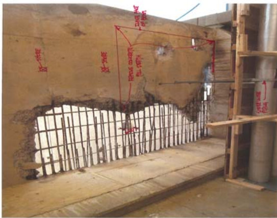
Regents Hall / Student Union Bridge repairs in progress and the stress crack in the south wall of Regents Hall prior to repairs
