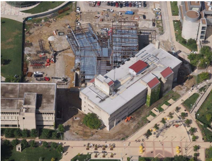
Aerial Photo of Construction Site - 2
