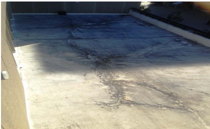
Current condition of the roof
